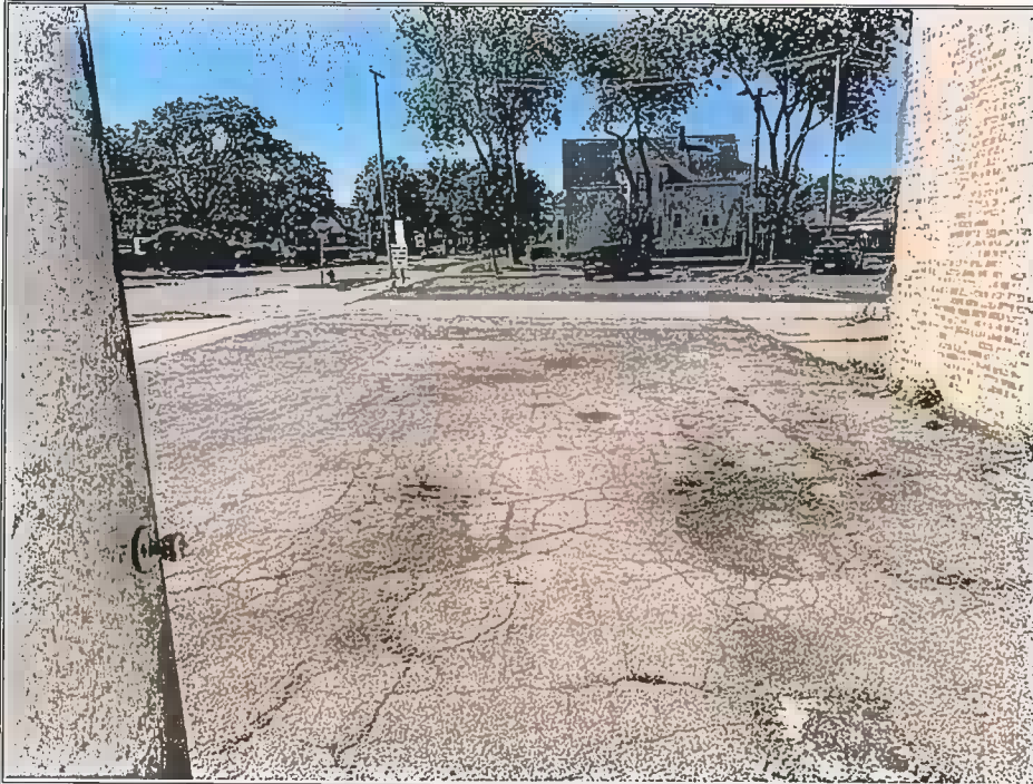
REAR PARKING LOT
