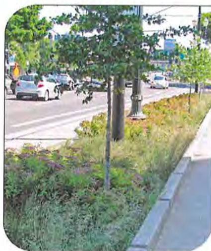
Stormwater garden curb extension Source: City of Grand Rapids
