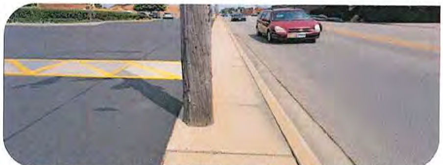
Several sections of sidewalk have obstructions that block the pedestrian access route. Public Right-of-Way Accessibility Guidelines state sidewalk segments must be 4 feet wide, clear of obstructions (IDOT guidelines call for 5 feet-wide sidewalks, 7 feet-wide if the sidewalk is on the back of a curb). If the sidewalk is less than 5 feet wide, passing spaces rules apply.
