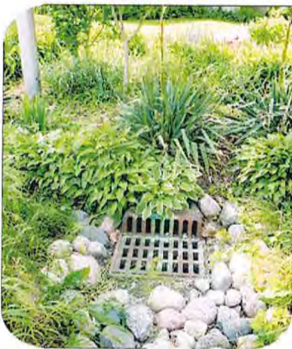
Green storm drain Source: CMAP
