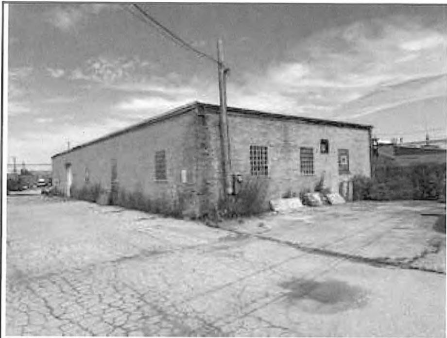
SOUTH AND EAST ELEVATIONS
