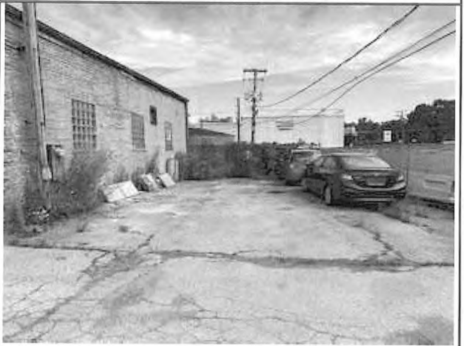
REAR PAVED AREA BEHIND BUILDING
