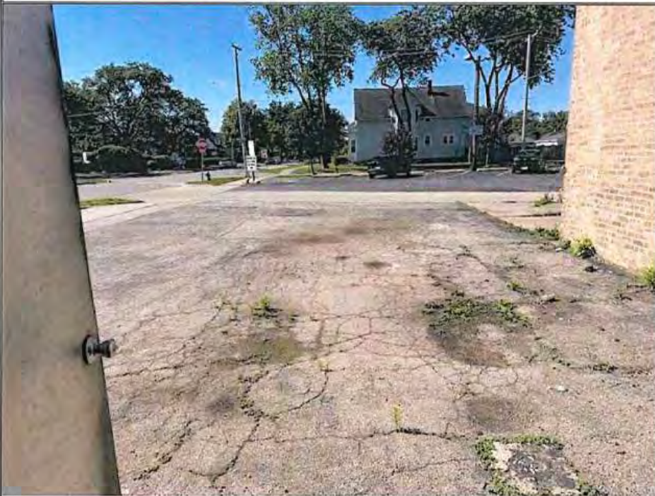
REAR PARKING LOT
