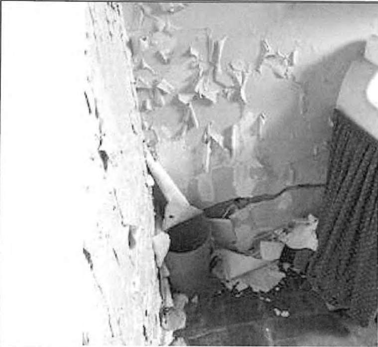
WALL IN WASHROOM
