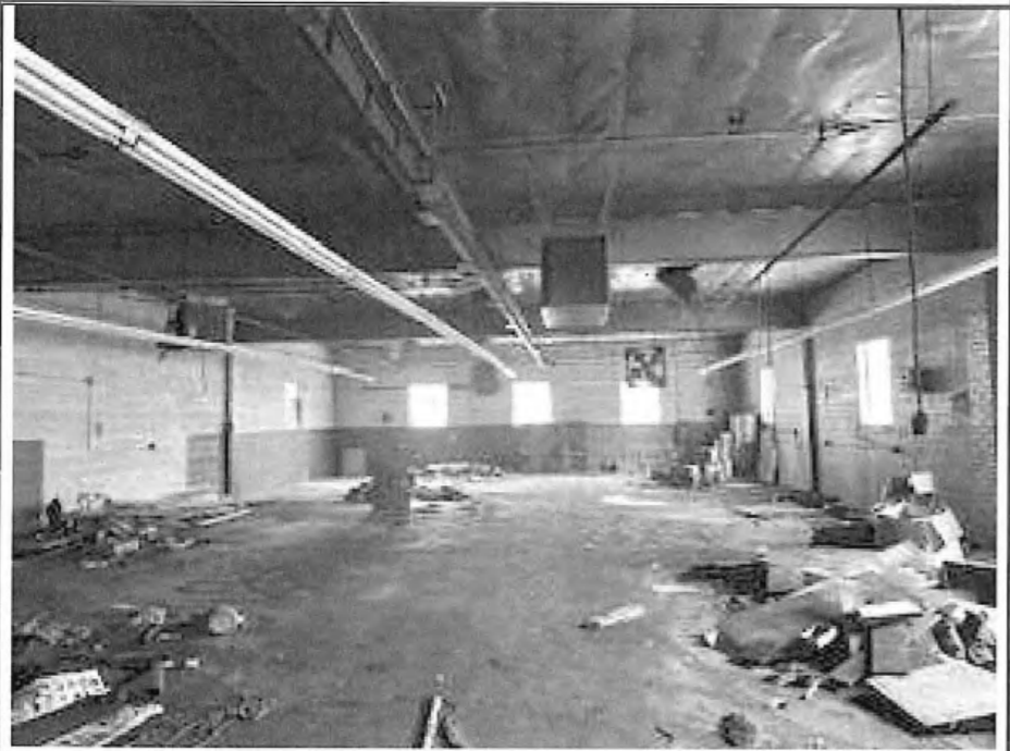
VIEW EAST ACROSS WAREHOUSE / SHOP AREA
