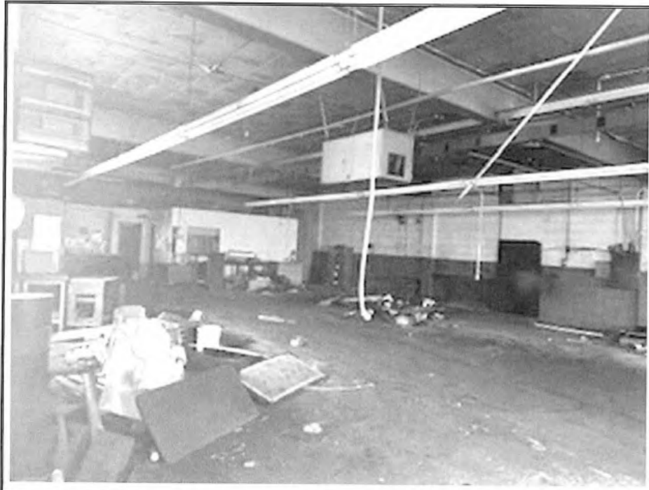
VIEW LOOKING NORTHWEST ACROSS SHOP AREA
