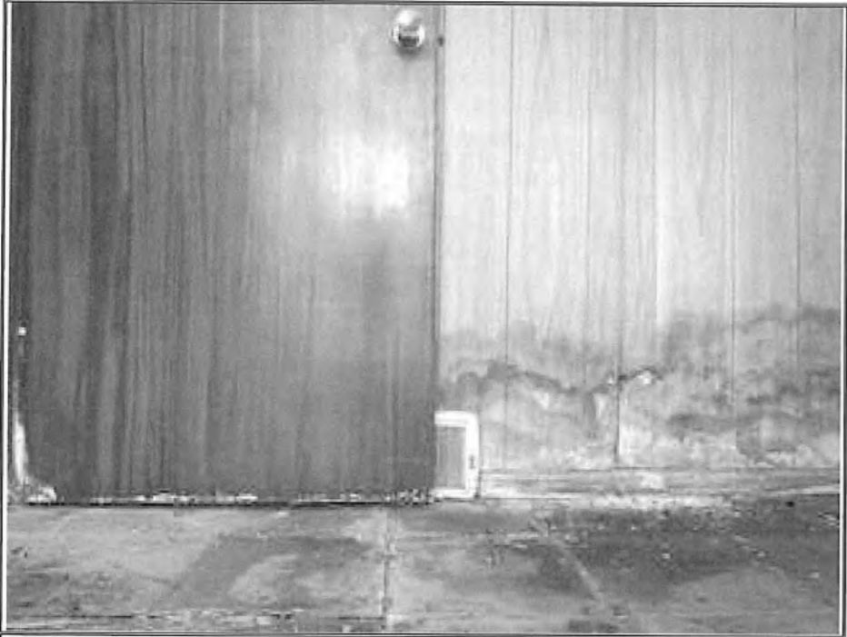
FLOOR AND LOWER WALL DETAIL IN OFFICE AREA
