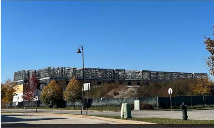
Construction is ongoing at 2900 Mannheim Road
