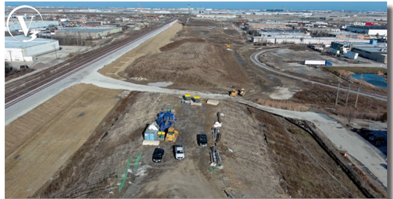
Future I-490 Corridor through the Village of Franklin Park Looking North.
