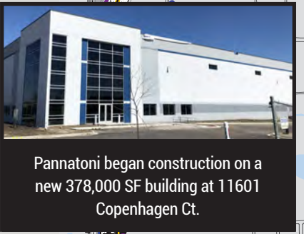
Pannatoni began construction on a new 378,000 SF building at 11601 Copenhagen Ct.
