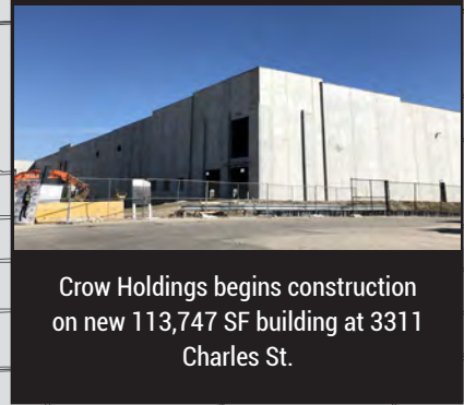
Crow Holdings begins construction on new 113,747 SF building at 3311 Charles St.
