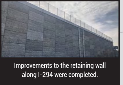
Improvements to the retaining wall along I-294 were completed.
