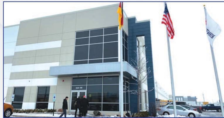
DB Schenker has moved into their new facility located at 10501 Seymour Avenue. The company is one of the largest integrated logistics Service Providers in the United States. Welcome to Franklin Park!
