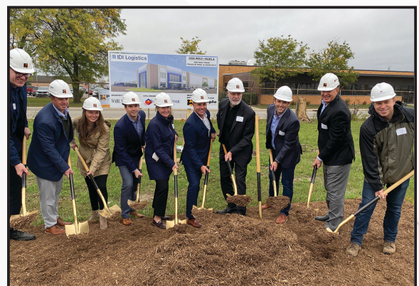
▶ Mayor Barrett Pedersen joined IDI Logistics in October to break ground on a 100,463-square-foot industrial building they are developing at 3500 Wolf Road.
