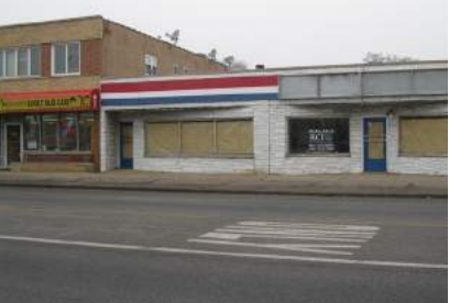
Commercial buildings along Grand Avenue
