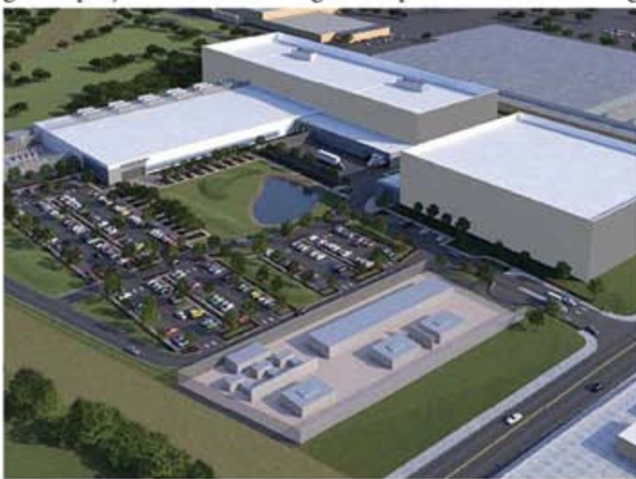
Digital Realty is investing several hundred million dollars in a state-of-the art data center in Franklin Park. The Village was recently awarded a grant to help the Village plan for the continued long-term growth and development of the community.
